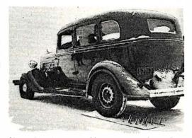
Photo taken after car was driven at 50 m. p. h. speed over spikes. Ordinary front tire blew out, but special tube in rear did not. Floating inner chamber is immune to punctures.
