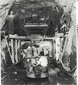
In "grasshopper" method of controlling traffic in tunnels, empty cars are swung overhead while loaded train moves out.
