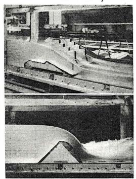
Lorenz A. Straub, University of Minnesota engineering professor, designed the above glass experimental cage for testing actual dams in miniature. Squares on the side of tank are used in graphing course of water over model.
