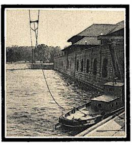
Above boat is powered from an overhead trolley and is used to keep floating refuse from entering power-house turbines.
