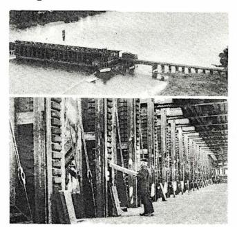
Top photo reveale an oddity in bridges spanning the Misaissippi. This unusual bridge can be swung around so allow passage of river boats or closed to permit trains to cross. Lower—Bridge tender removes a wooden plank from one of a long row of rail supports to compensate for rising river.
