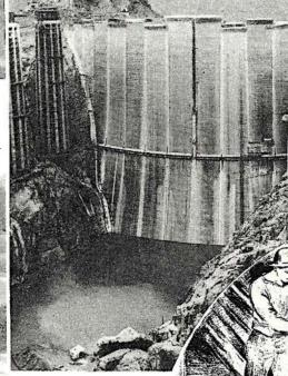
bowering of this 3,000,000-pound steel door closed first of Colorado river diversion tunnels, marked beganning of huge reservoir which will extend 115 miles upstream, flooding area of 227 square miles. Photo at right shows water level rising behind massive Boulder Dam. Intake towers on either die will eventually be submerged, and then supply water for the power generating plant.
